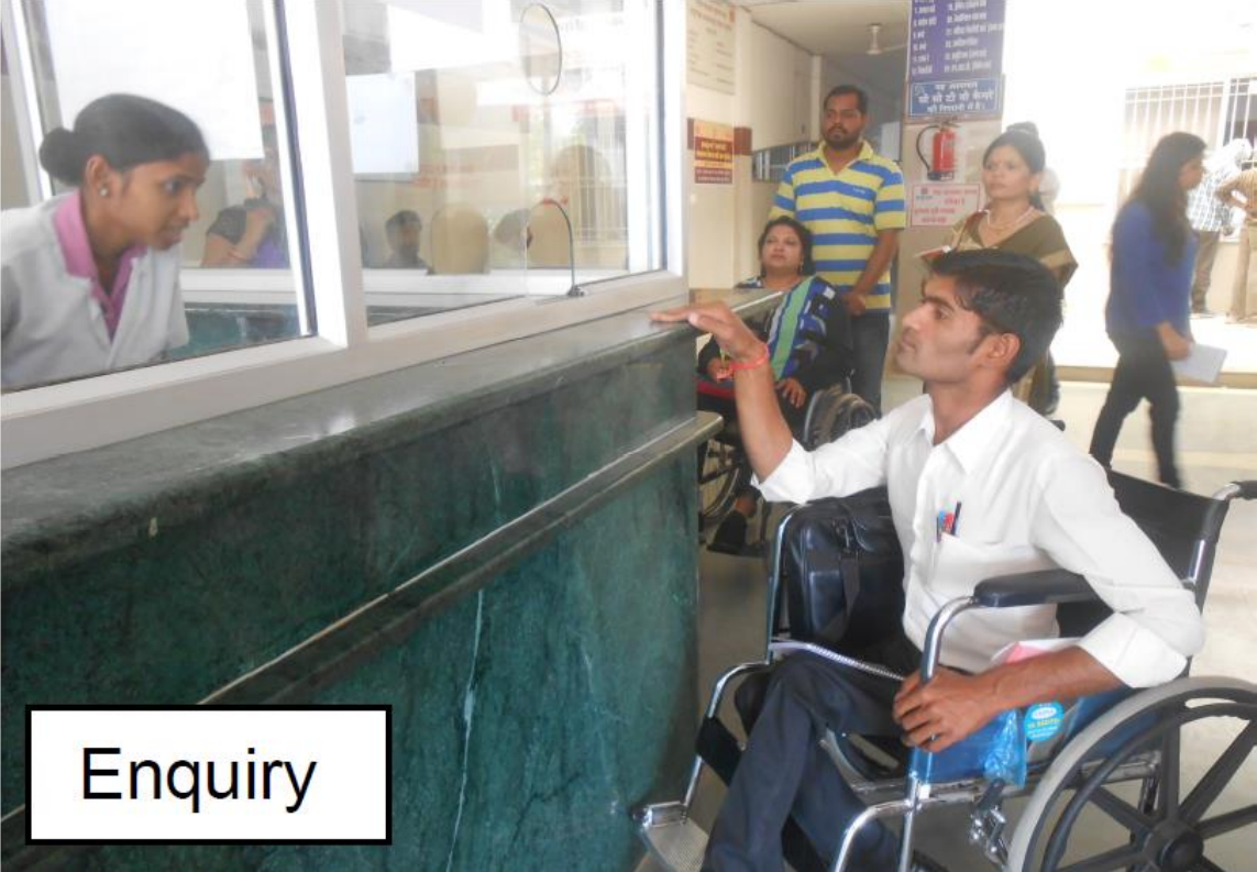
Figure 1. The enquiry counter at CHC Kolar Road vision centre is not accessible, being at a height of 1120 mm, with a communication opening at 1550 mm.
